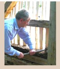
Mud and Stud, a vernacular form of wattle and daub, comprises a mixture of earth, clay, straw water being in-filled within a lightweight timber frame with laths and traditionally having a thatcl roof. It is peculiar to Lincolnshire, and versions of it can be found all round the world. Such buildings have links to Tennyson through the village of Somersby in the Lincolnshire Wolds, ar Jamestown, the first permanent English settlement in the Americas.
